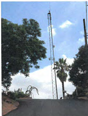
80 ft. Communication Tower Above Main Office
