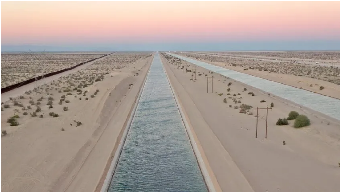
The San Diego County Water Authority upgraded the All-American Canal in Imperial County to reduce reliance on the Metropolitan Water District. Courtesy of the authority
