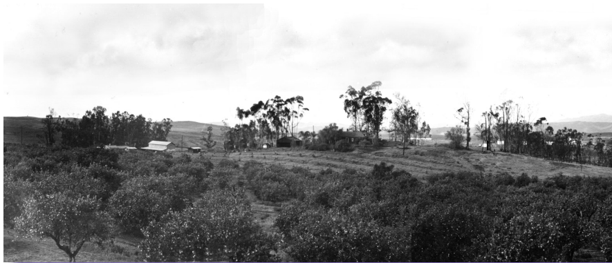
Water Reclamation Plant on Alturas Road, before Camp Pendleton. Photo courtesy of Tom Rodgers, (1922)
