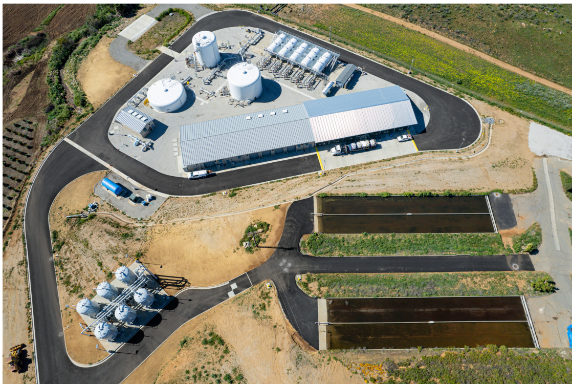
Santa Margarita Groundwater Treatment Plant
