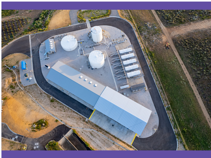
Aerial View of the SMGTP
