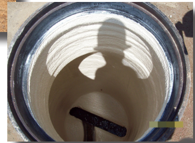
Pipeline relining program
