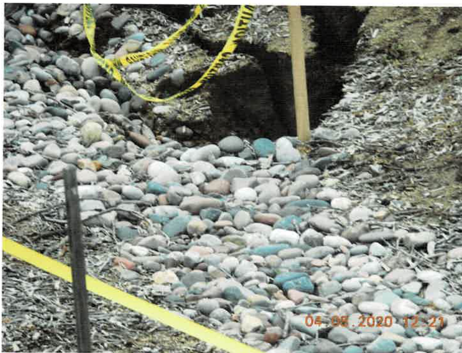
April 8, 2020 Hole has expanded due to rain. Taken on Wednesday April 8, 2020.
