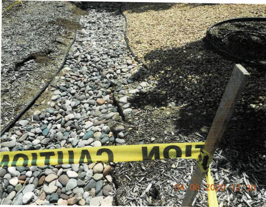
Sinking continues toward back of lot toward Stage Coach Lane. Approximately 50 feet from Inlet on Palomares Road Apr 8, 2020
