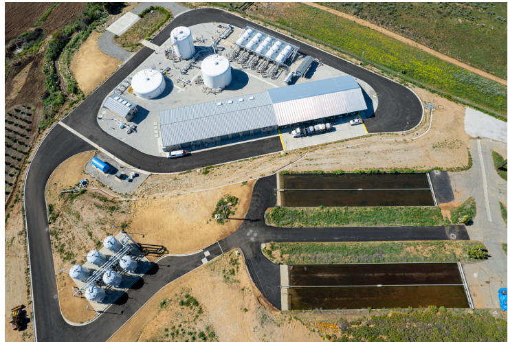
Santa Margarita Groundwater Treatment Plant
