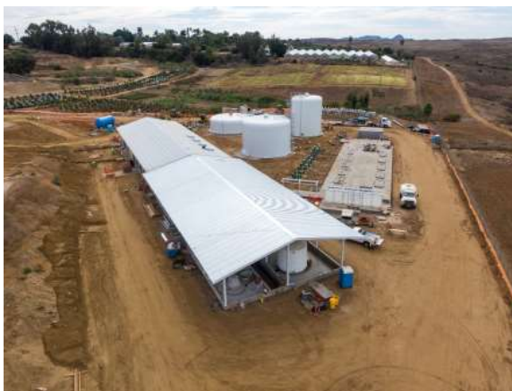
Construction progress of the SMGTP
