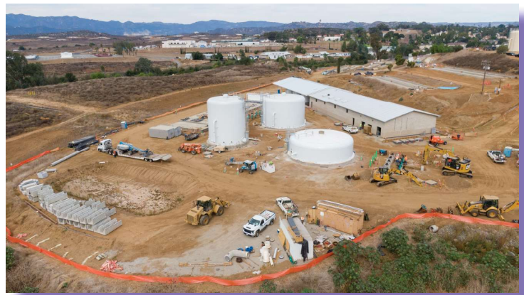
Construction progress of the SMGTP
