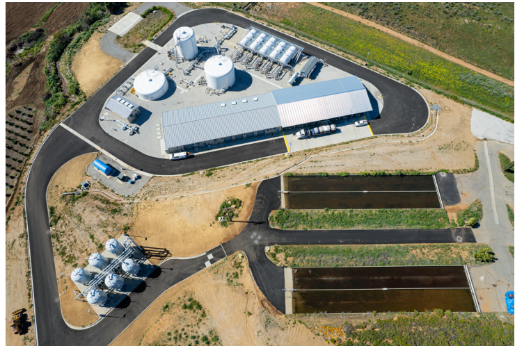
Santa Margarita Groundwater Treatment Plant
