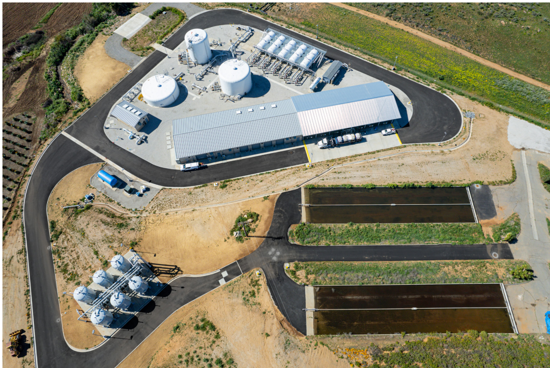
Santa Margarita Groundwater Treatment Plant
