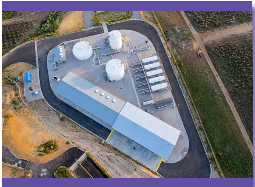
Aerial View of the SMGTP
