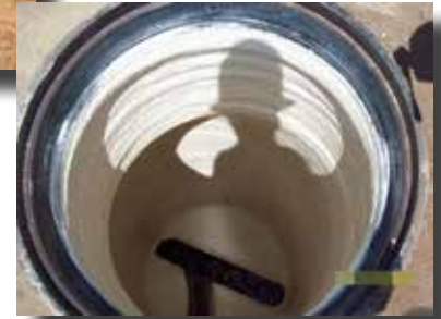
Pipeline relining program
