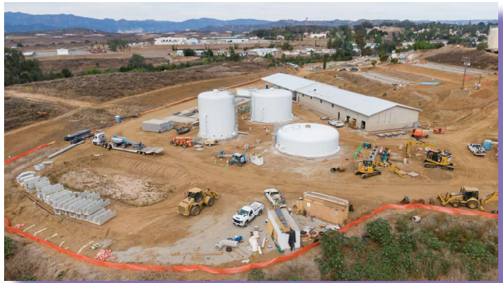
Construction progress of the SMGTP
