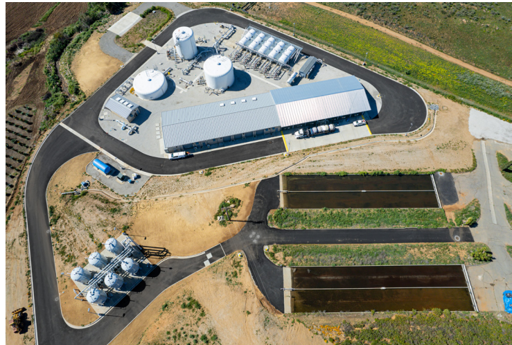
Santa Margarita Groundwater Treatment Plant
