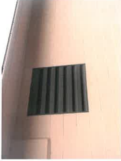
16. View of wall vent in aeration blower building. 1/2 inch wire mesh is placed behind the louvers.
