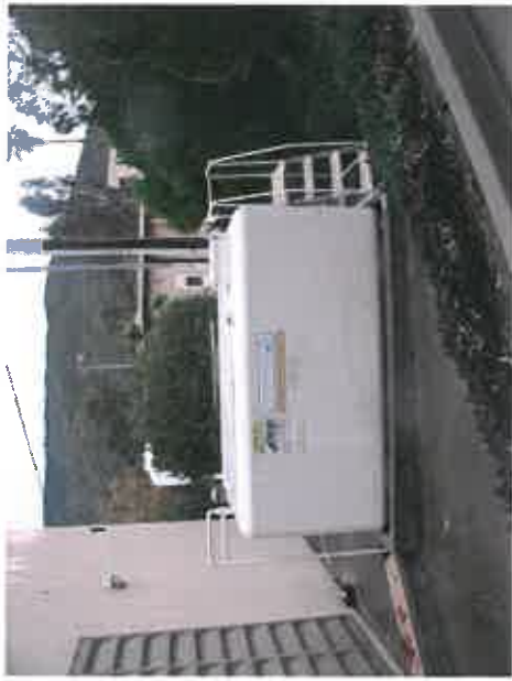
41. View of Diesel Tank near Generator Building. Tank is a ConVault type tank.
