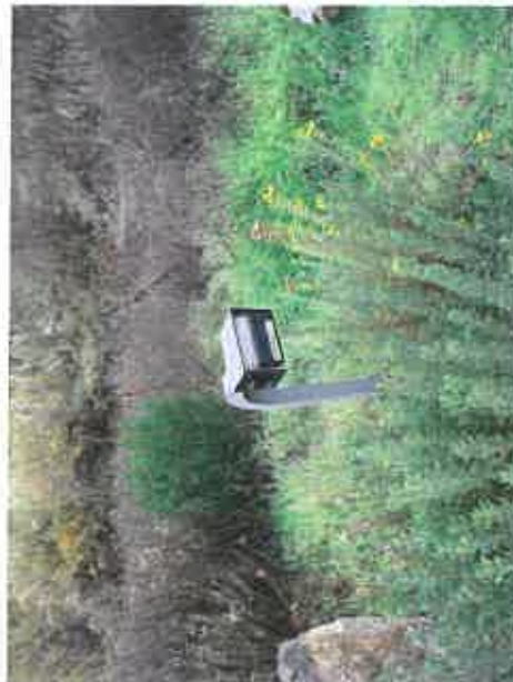
61. View of controller for automatic gate including Knox key access for fire department.
