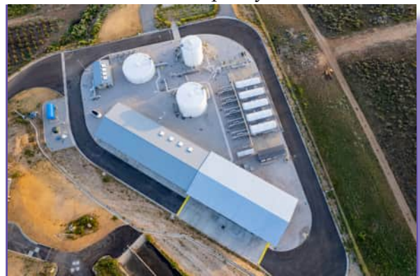
Aerial View of the SMGTP
