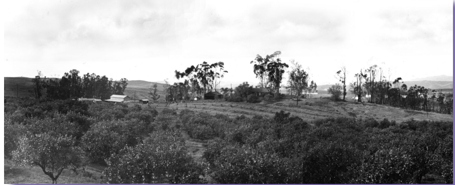
Water Reclamation Plant on Alturas Road, before Camp Pendleton. Photo courtesy of Tom Rodgers, (1922)
